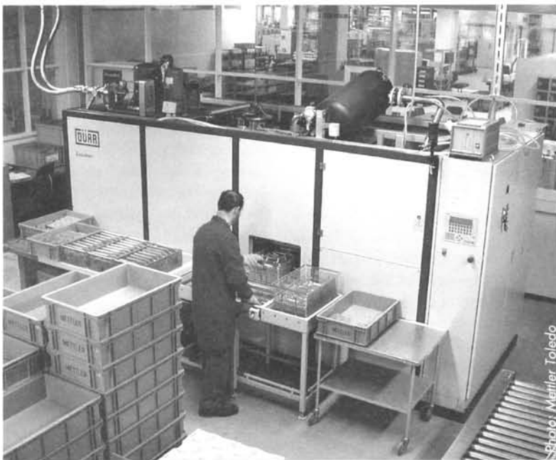
Improved cleaning quality, less harm caused to the environment and a significant increase in the efficiency of the entire cleaning process – the results of Mettler Toledo's installation of a new hydrocarbon plant.
